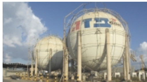
Petrolgas Group, ISRAEL Petrolgas group is active in the areas of petroleum and construction. Together with Pazgas they control 40% of Israel's domestic gas market and turnover in excess of $1 billion annually.
