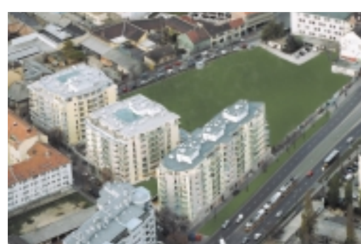
EUMOR, Budapest, HUNGARY Central Park 860 housing units and 7,500 sqm of commercial area.
